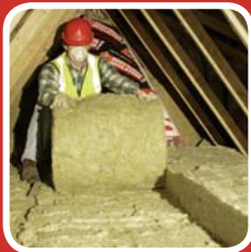
Roof insulation
