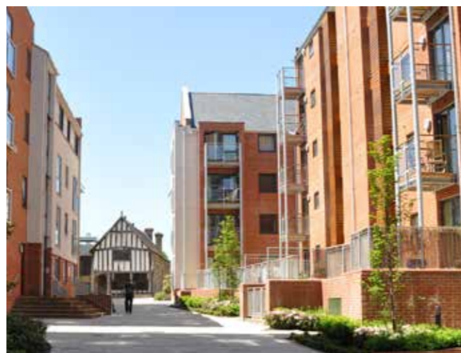
3 Brewhouse Lane is an example of a once lost route, now re-established as part of a recent city centre development proposal
