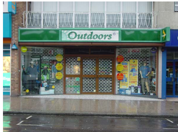
A well-designed security shutter that protects the shop's stock but retains a window display, allows views through into the shop and lets light spill onto the pavement.
