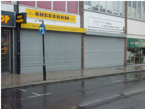
Shutters should be internal, and of the open lattice type, to avoid blank frontages predominating at night.
