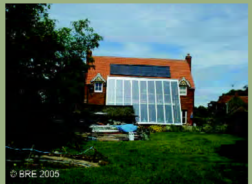
Dwelling fitted with solar water heating panels and large south facing conservatory for passive solar gain © Bre 2005
