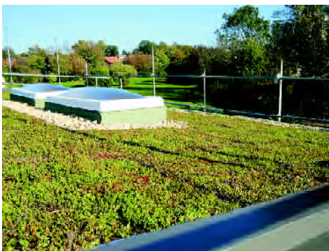
A green roof with sedum planting used on a public toilet block at Weston Shore, Southampton, designed by Southampton City Council Building Design Services
