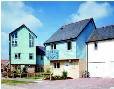
Ecohomes - award winning energy efficient housing; a joint venture project between Countryside Properties and SEEDA, St Mary's Island, Chatham Maritime, Kent - Developer: Countryside Properties Architect: Countryside Properties Architects with OSP Architecture © Countryside Properties
