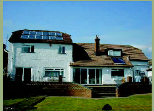
Dwelling fitted with solar water heating panels (right) and photovoltaics to the roof © Bre 2004
