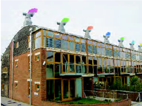
Energy efficient housing that incorporates passive solar gain and photovoltaic cells, amongst many other features - BedZed
