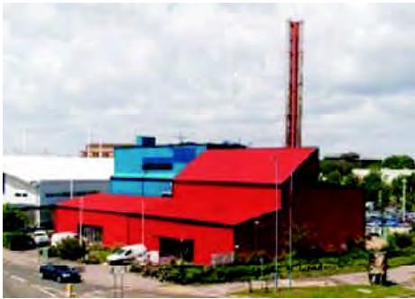
The Utilicom combined heat and power plant in Southampton © Utilicom Ltd
