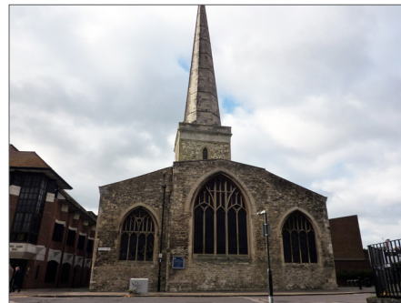
A. View looking west along Bernard Street to St Michael's Church, c1890 (copyright) Historic England B. Present day east facade
