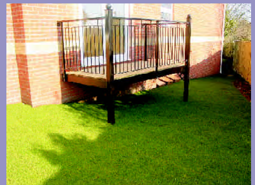
Balconies should not be provided at ground floor levels as the space below them cannot be easily maintained; a terrace would have been more appropriate here
