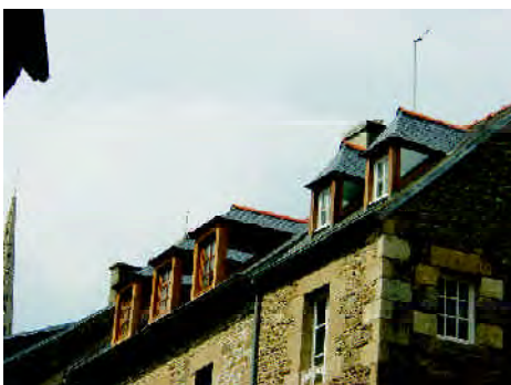
Dormer windows in Brittany, France, use a simple construction allowing the sides to be glazed
