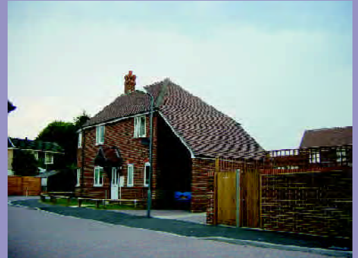
This carport has been sensitively designed using an extension of the main roof at the same pitch and with the same roof tiles
