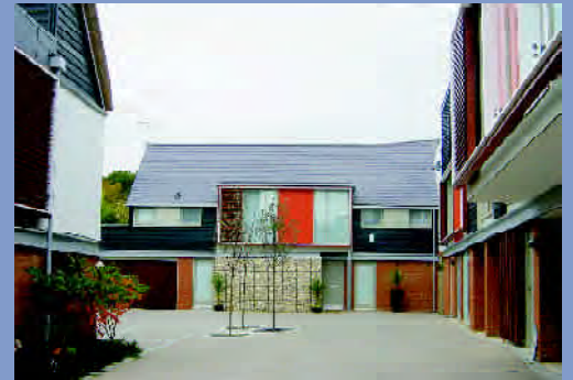
The use of shared surfaces and soft landscape can create an attractive courtyard setting - Harlow
