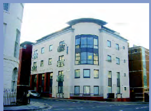
This good example of an inner city apartment block illustrates how setting back the elevation on the corner and slightly raising the height can add interest to the development. The development also respects the scale and proportions of the Georgian buildings opposite - Portland Street, Southampton
