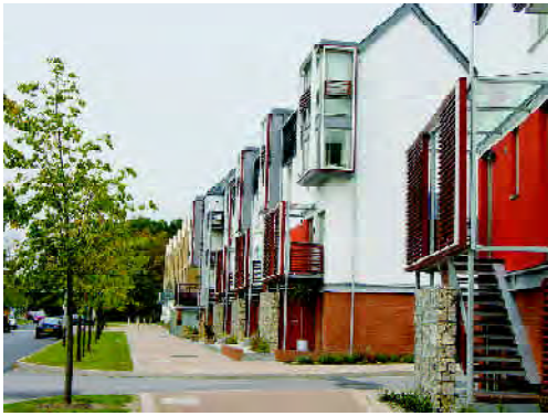
The line of street trees and well defined frontage to this new housing development frame a distant view of woodland - Harlow
