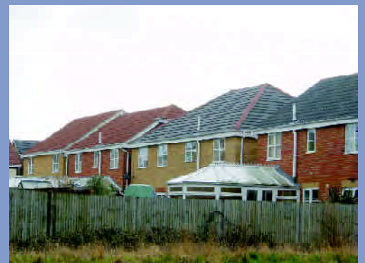
Exposed soil pipes to the rear elevations of these houses look unsightly
