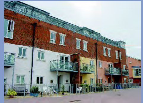
The use of brick at third floor level makes this development look top heavy, however the use of galvanised steel is a sensible choice in this waterside location - Hythe
