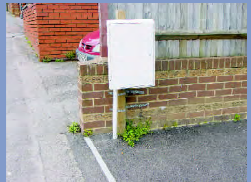
Meter cupboards should not be located in visually obtrusive places and where they are vulnerable to damage
