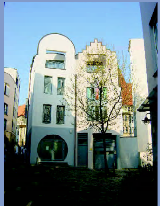
A contemporary take on traditional housing creates an attractive new focus for this courtyard - Bremen
