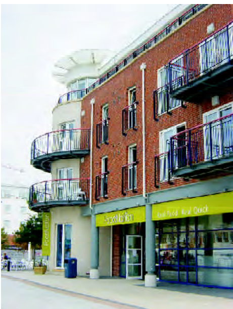
The corner of this building is emphasized by a change in elevational treatment, balconies and a taller roof feature - Portsmouth
