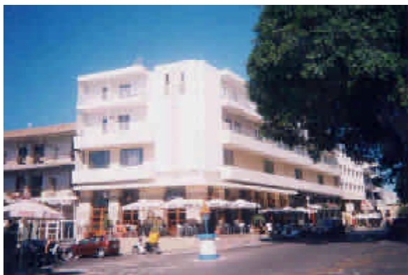
Cafés, shops, and commerce can all sit comfortably with one another even in one building on different floors, providing life to the street and the services required to sustain adjacent city living, as in this example in Rhodes
