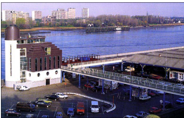
Marine inspired architecture providing a distinctive landmark on the waterfront Zuiderterras Cafe, Antwerp
