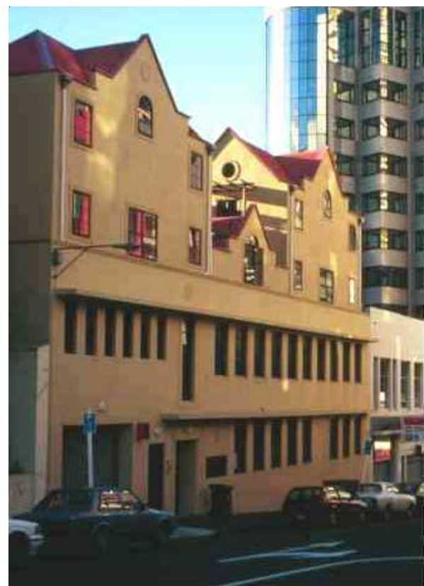
Residential infill above a car park in Auckland.
