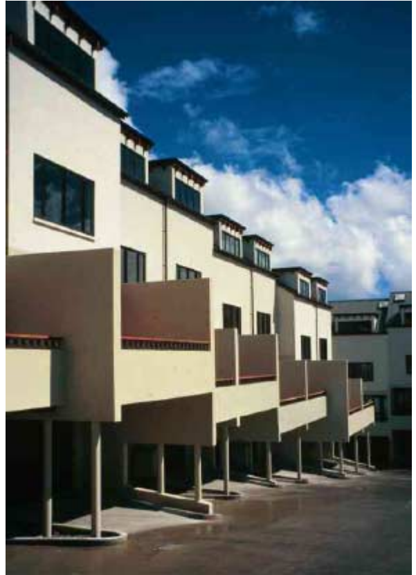
Terraced townhouses with undercroft parking at rear - Auckland.
