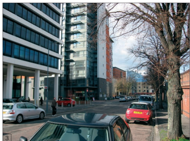
01 View east along Richmond Street (Mercury Point in the left and Richmond House on the right) 02 The architecturally distinctive Mercury Point 03 The public realm of College Street
