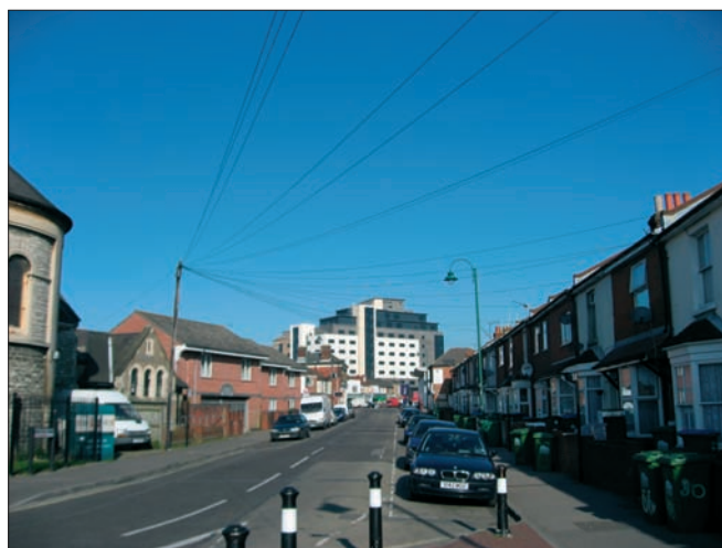
View looking north along Brinton's Road to Charlotte Place
