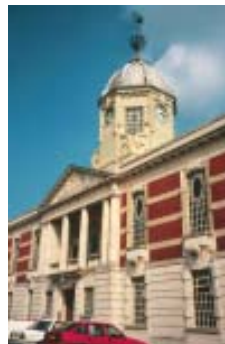
Harbour House, Town Quay Southampton
