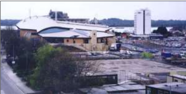
The vacant West Quay Phase 3 site will provide a new landmark public space
