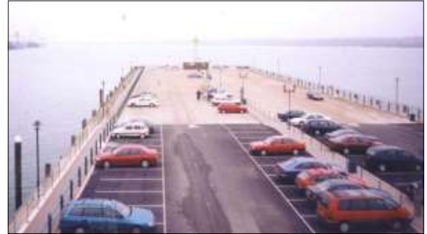
The piers along the waterfront, including Town Quay, offer magnificent opportunities to locate new landmark buildings and public spaces
