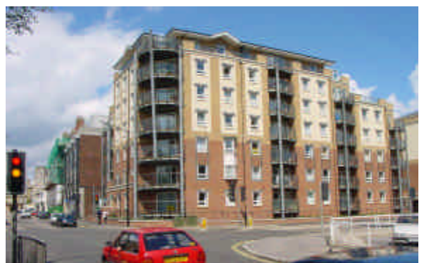
Merchants' Quarter: a recent residential development within the Old Town, which reinstates historic alley-ways through the site, but whose massing and scale could be more sensitive to the Old Town's character
