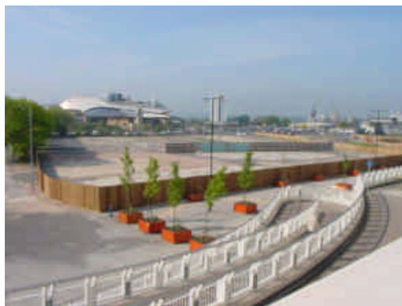
The West Quay Phase III development site to the northwest of the Old Town, which, amongst other things, promotes the creation of a City Plaza for major events. From within the Old Town, these will be able to be viewed from the top of the Town Walls, which stand some 20ft high
