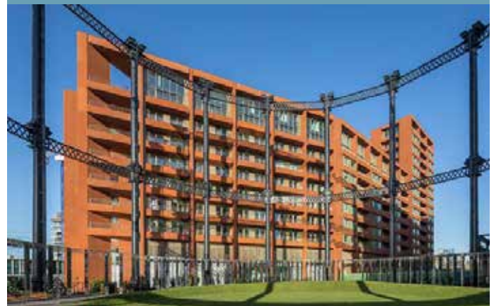
Tapestry Building, Kings Cross - Mixed-use Energy Centre
