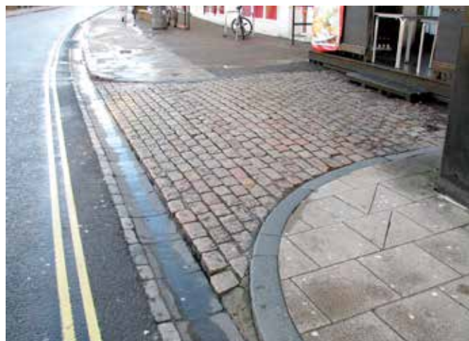
Fig 30 Pavement crossover and black gutter gullies
